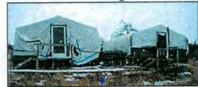
Photo 10 Buildings G and H
