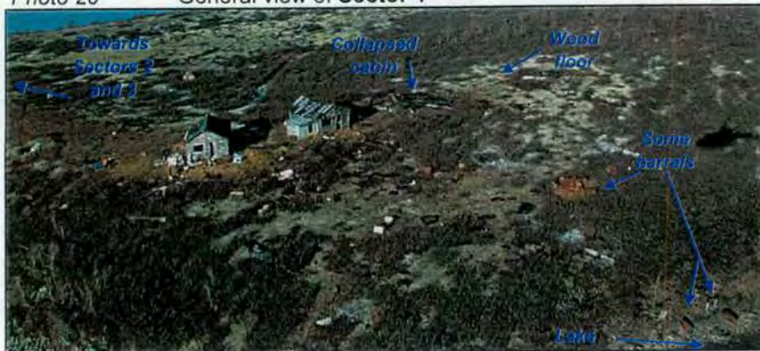
Photo 20 General view of Sector 1
